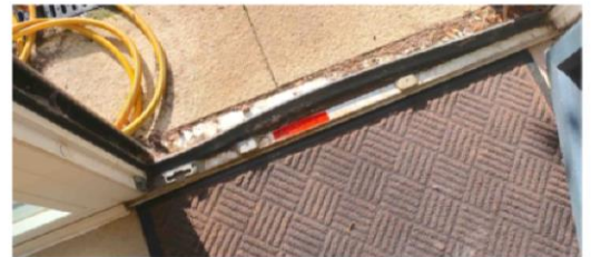
FIGURE 6 (above) Back door cill with detached weatherstrip, bowing outwards in the middle.
