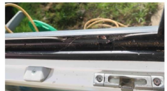
FIGURE 7 (right) one of two folds in the draught seal of the window to the left of the back door
